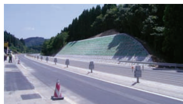
のり面防災対策
