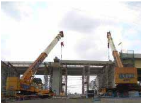
(橋梁修繕の実施例)
