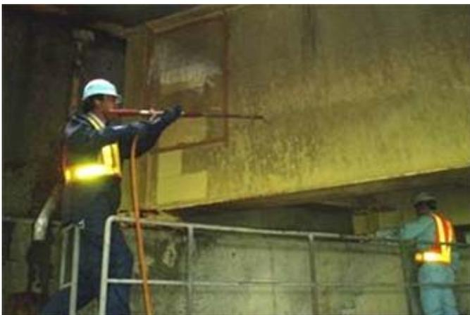
桁端部塩分洗浄状況
