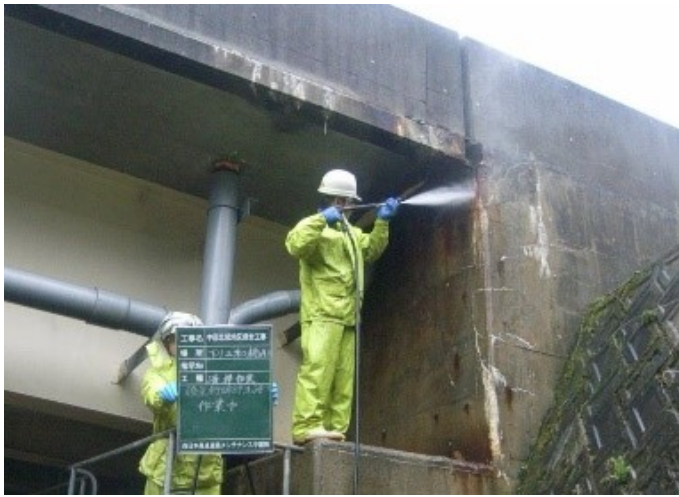
桁端部塩分洗浄状況
