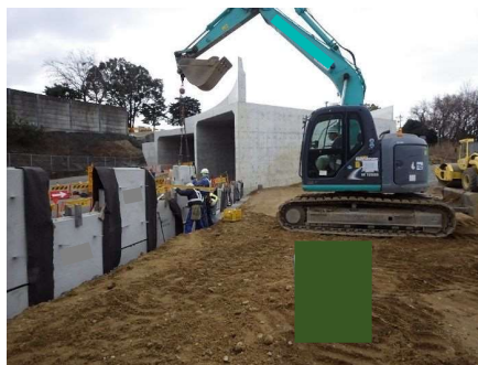
壁面材組立て
