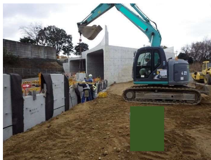
壁面材組立て
